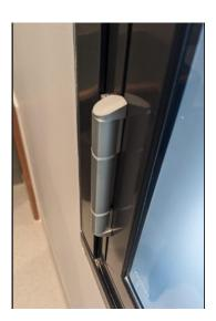
There are inconsistant gap between the purpose built anti-ligature hinges located in bedrooms. The gap can potentially be used to loop a cord or other materials over the hinge and could trigger a self-harm incident e.g. the cord from surgical masks looped over the hinge for self-harm.
